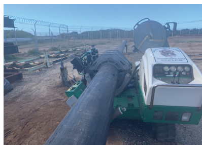
HDPE Fusion Equipment and Training
